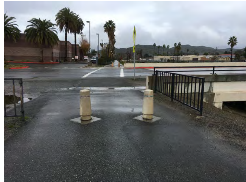
Bollards restrict vehicular access to multi-use facilities, such as above, ensuring safe separation of modes while allowing emergency access when needed.
